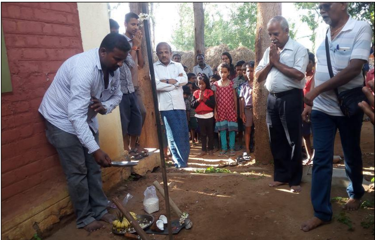
Start of work on Boys' dormitory on June 3 rd 2017
