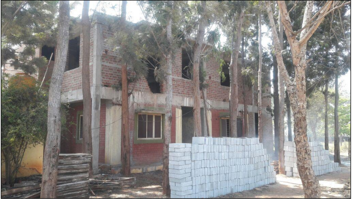
Boys Dormitory as on 20 th Feb 2018
